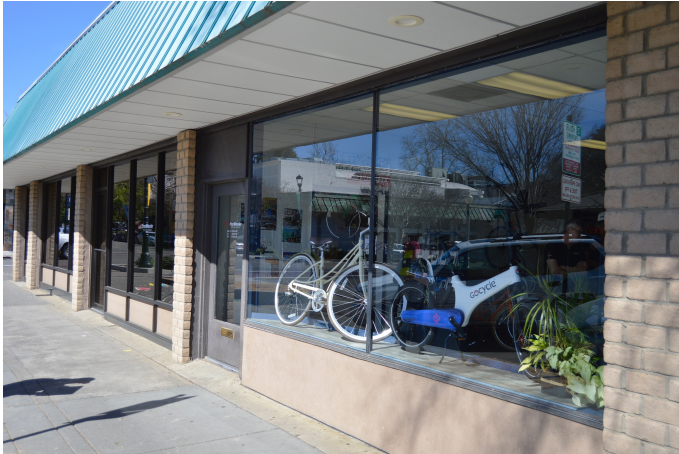
Figure 1. Storefronts along south elevation with opaque base panels (left), and one storefront with a stucco-covered bulkhead (right), looking northwest.
